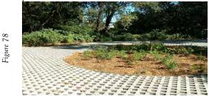
**Grass pavers** allow infiltration of stormwater while providing a load-bearing surface. This picture shows the project in the final stages of completion. The voids between the concrete lattice structure should be filled with a loamy material to allow for sufficient infiltration rates.
