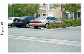
*Parking lots* should collect and drain in a single swale
