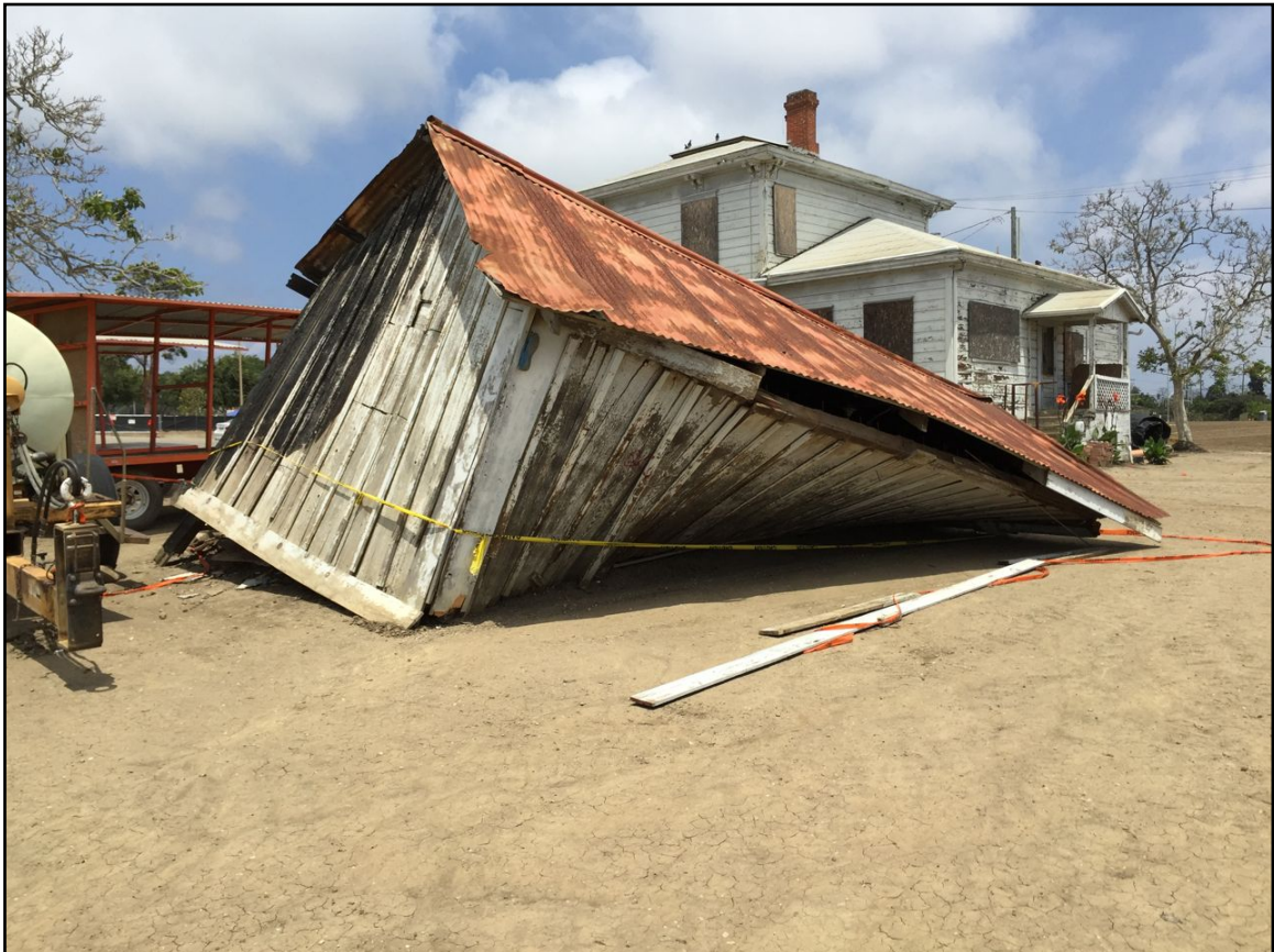
Photo 10. Garage 2, western and southern elevations. [23 July 2015]
