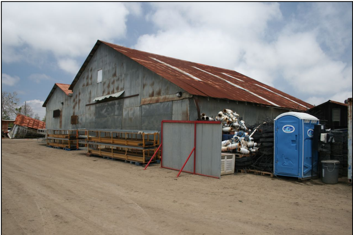
Photo 8. Metal barn, western and southern elevations. [23 July 2015]
