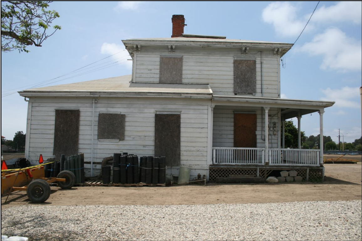
Photo 3. Main residence, side (eastern) elevation. [23 July 2015]
