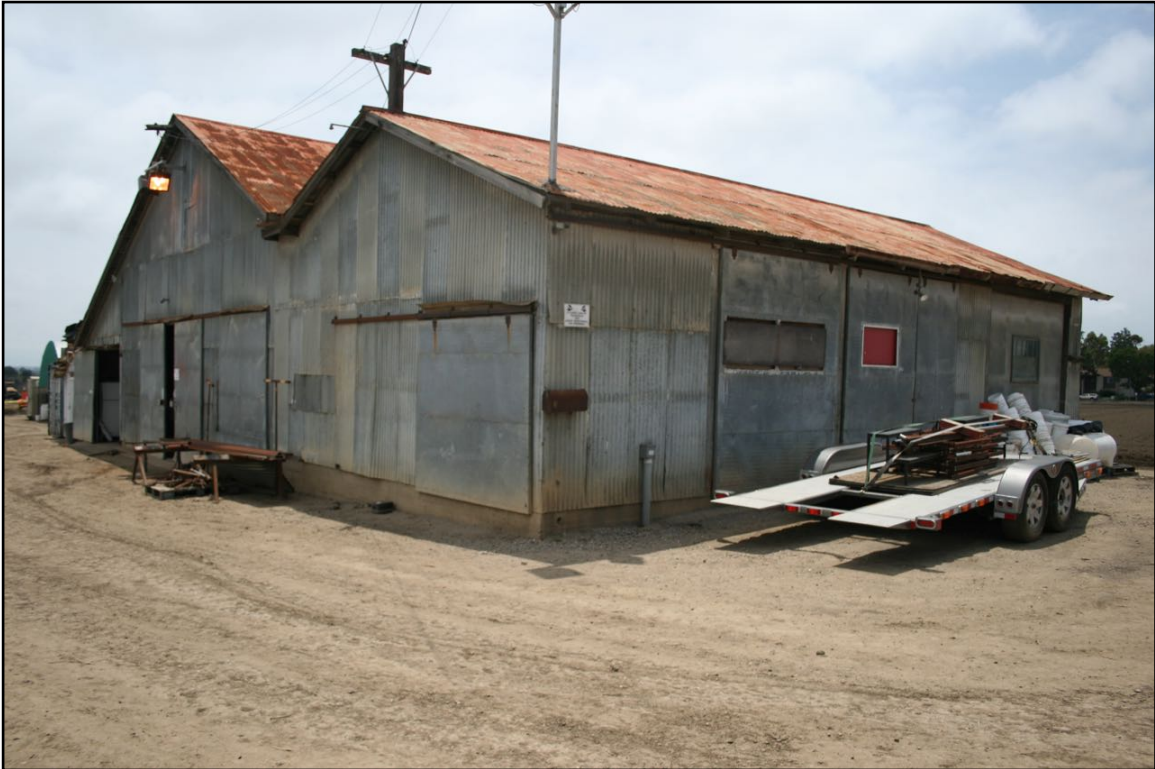
Photo 7. Metal barn, eastern and northern elevations. [23 July 2015]
