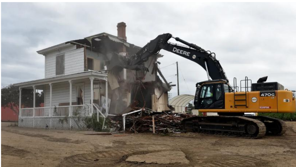
Figure 2 – Day Ranch House Undergoing Demolition, 2017
