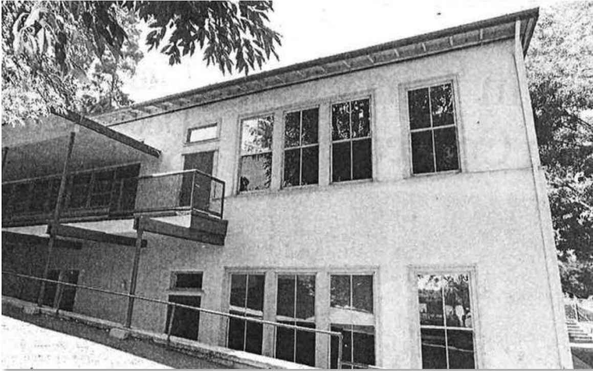
Figure 1 – Former Olivelihoods School Building, 2001
