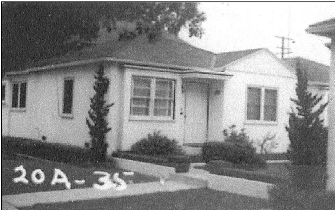
Photo 6. Unit 127, from northeast. Ventura County Assessor, c. 1955.
