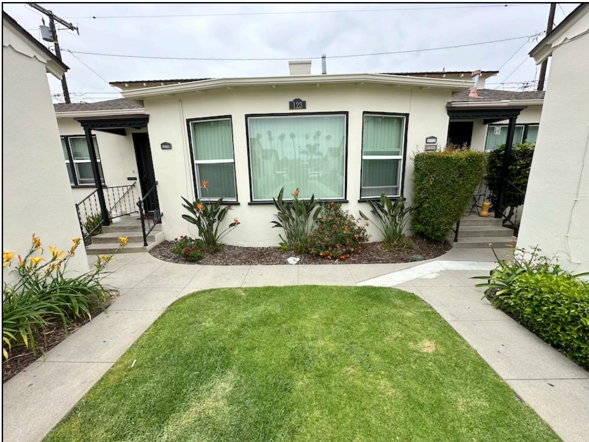
Photo 18. Units 123 and 123A, viewed from east. [5-15-2024]
