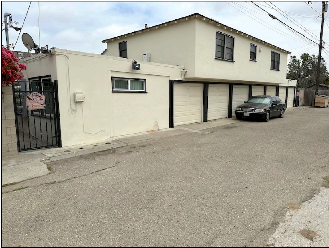
Photo 19. Rear of units 123 and 123A and garages, viewed from northwest on alley. [5-15-2024]
