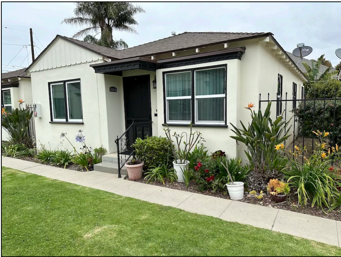
Photo 15. Unit 119A, viewed from southeast. [5-15-2024]
