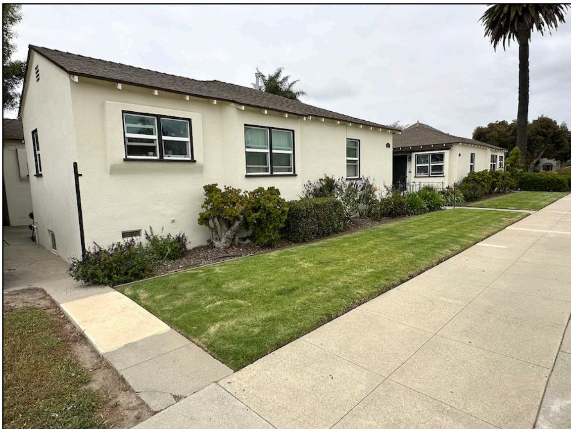
Photo 10. Street elevation, viewed from southeast. [5-15-2024]
