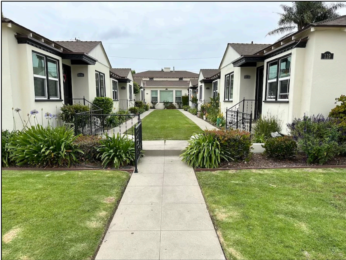
Photo 11. Courtyard, viewed from east. [5-15-2024]
