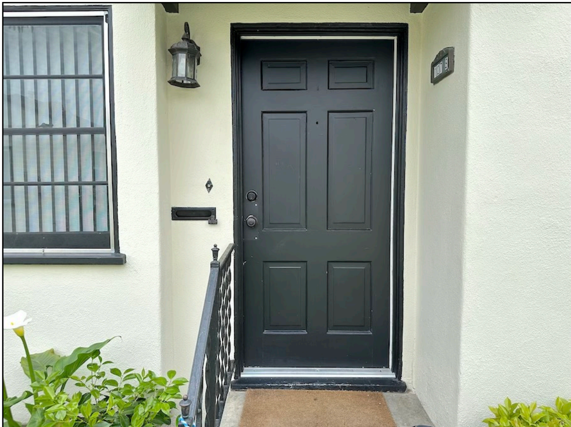
Photo 20. Entry door treatment for individual units, typical. [5-15-2024]
