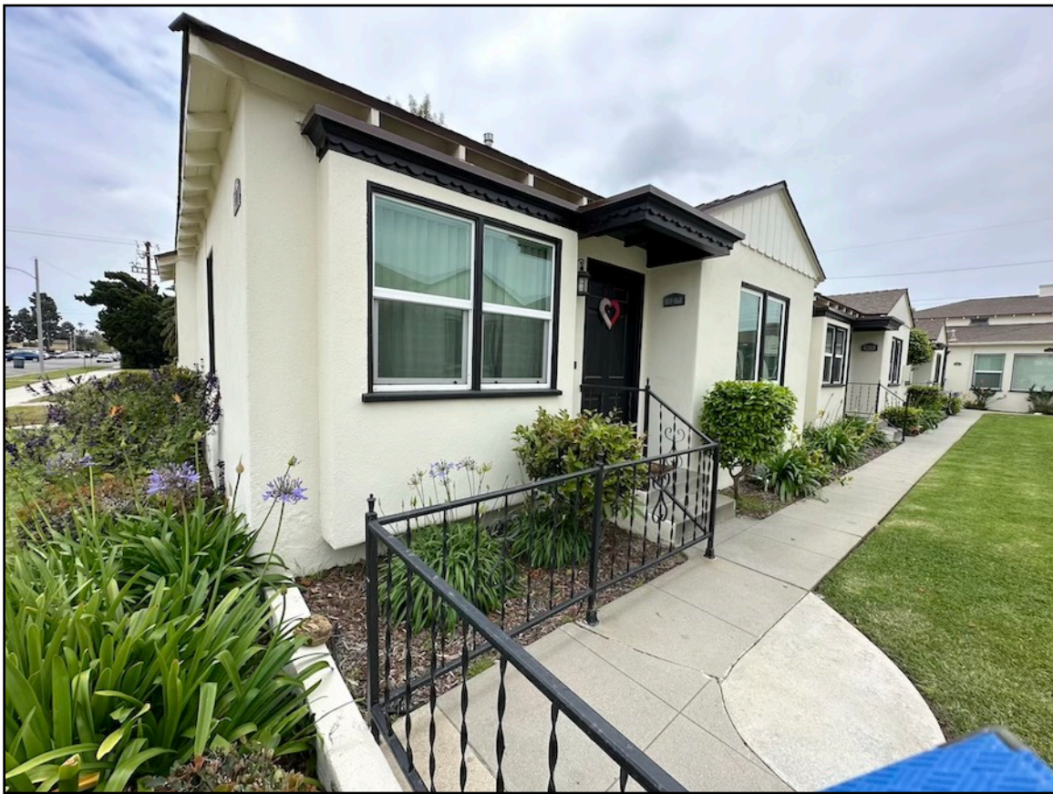
Photo 13. Unit 127, viewed from northeast. [5-15-2024]
