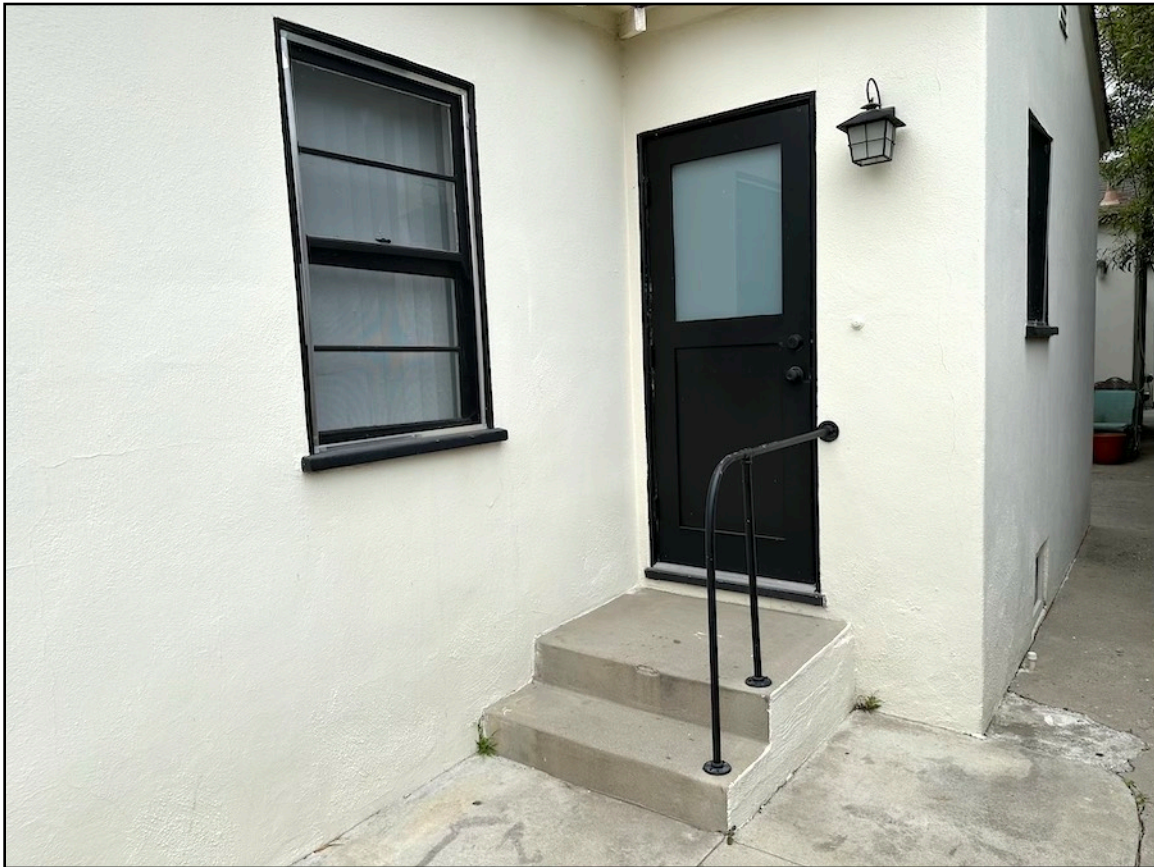
Photo 21. Rear stoop and door treatment for individual units, typical. [5-15-2024]
