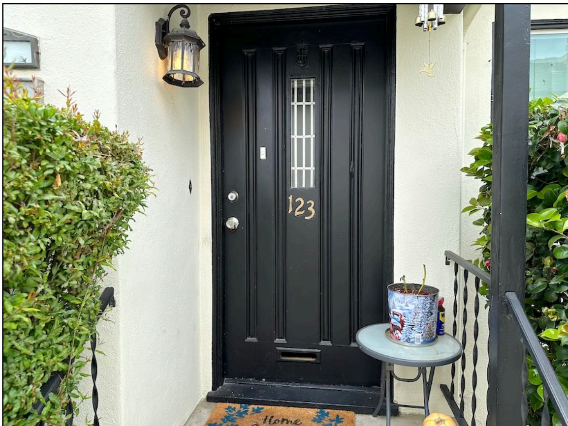
Photo 22. Entry door treatment for duplex units, typical. [5-15-2024]
