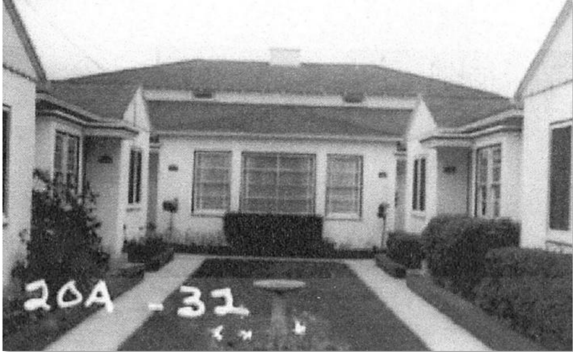
Figure 1 – Historical View of Subject Property, c. 1955
