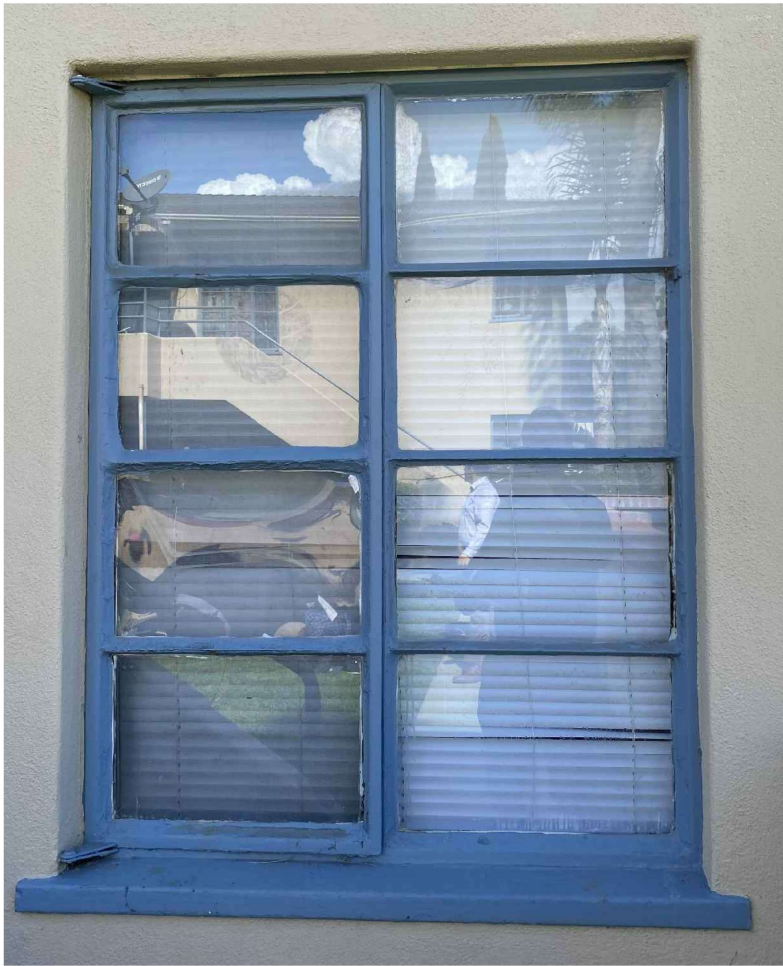
ORIGINAL STEEL CRANK OUT CASEMENT WINDOWS
