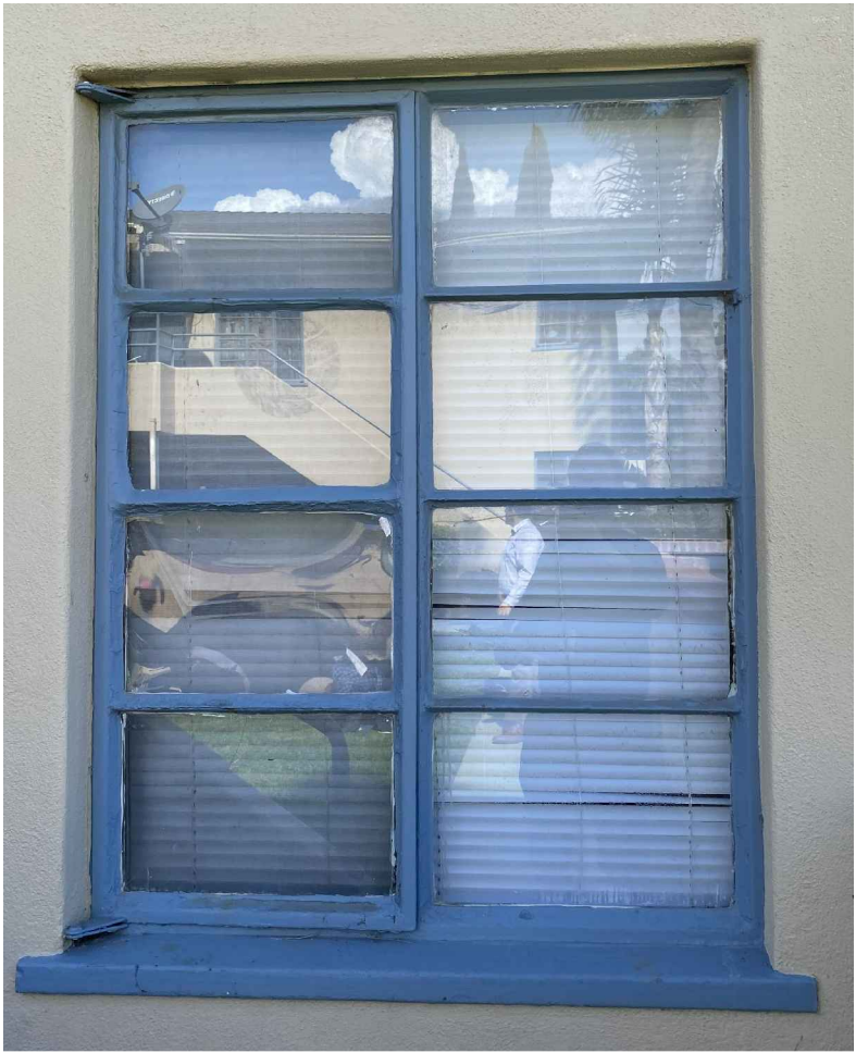
ORIGINAL STEEL CRANK OUT CASEMENT WINDOWS
