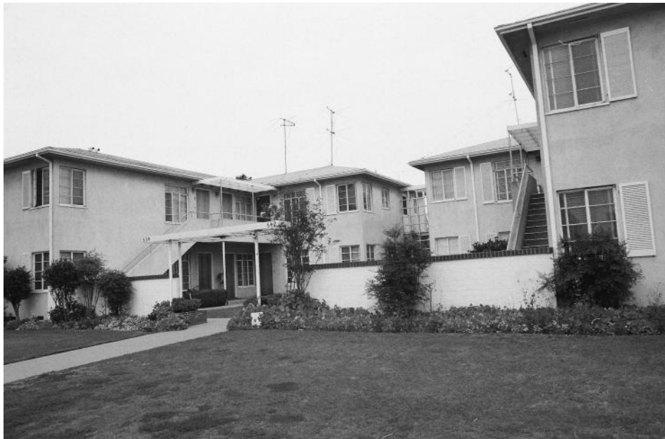
Figure 4 – Western elevation, showing original wall configuration, pergola, and screen (1981)
