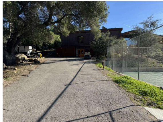
9. Existing Road on the North
