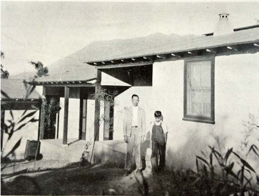
The newly-completed Chinese Quarters, now known as the Health Center. View looking west, 1932. Source: The Thacher Notes .
