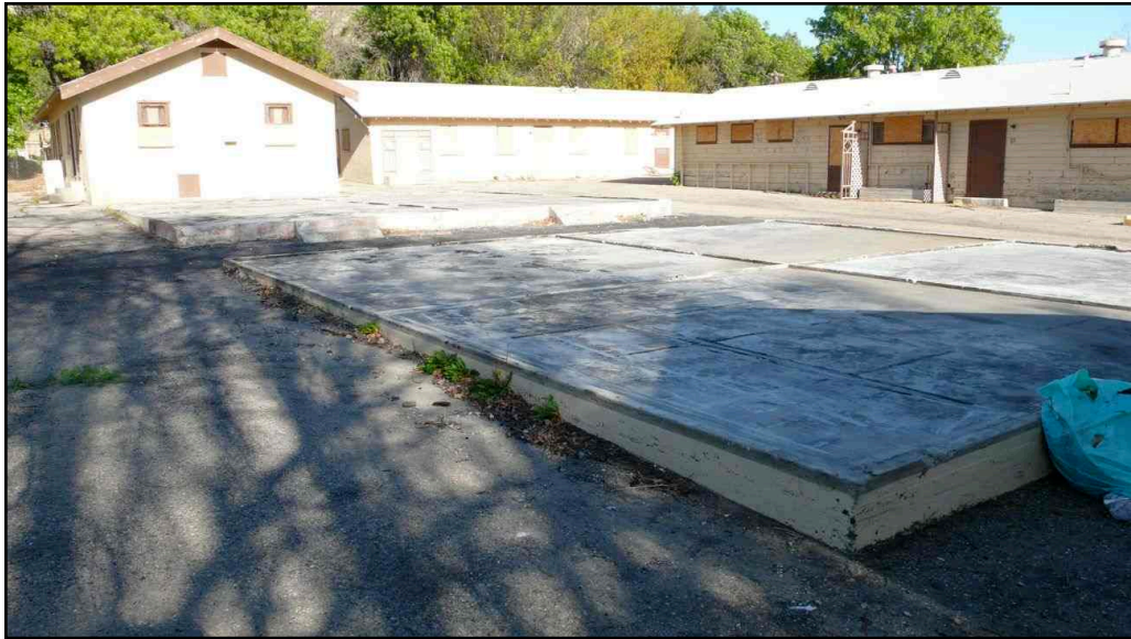
Photo 11. Foundations, facing north [16 February 2008]
