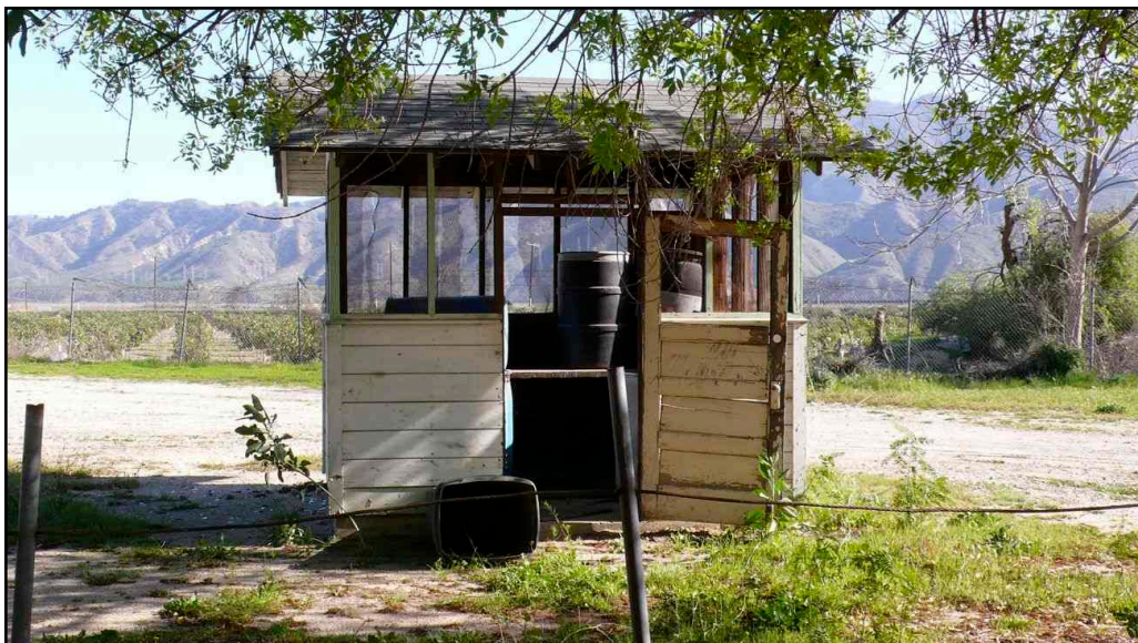
Photo 9. Trash enclosure building, western elevation [16 February 2008]
