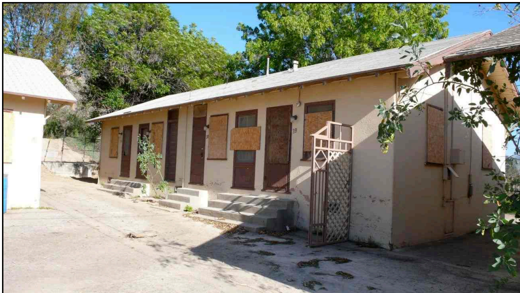
Photo 5. Bunkhouse, western & southern elevations [16 February 2008]
