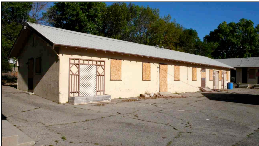
Photo 6. Bunkhouse, southern & western elevations [16 February 2008]
