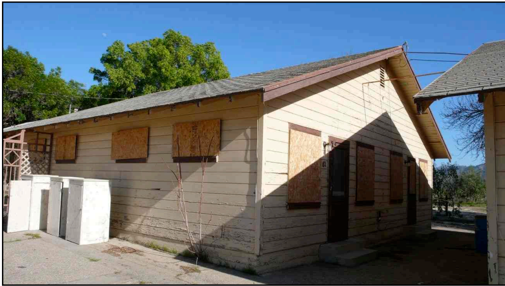
Photo 4. Bunkhouse, western and southern elevations [16 February 2008]
