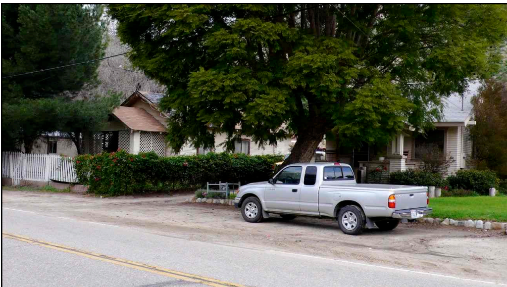
Photo 15. View across Center Street from project site, facing north [21 February 2008]
