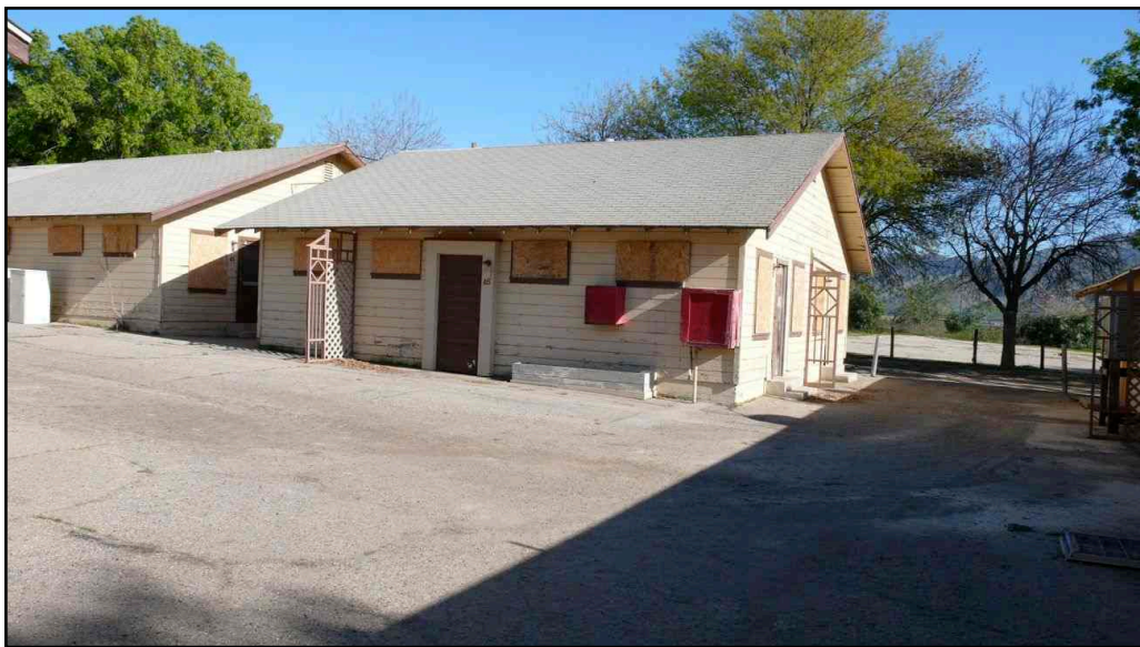
Photo 3. Bunkhouse, western elevation [16 February 2008]
