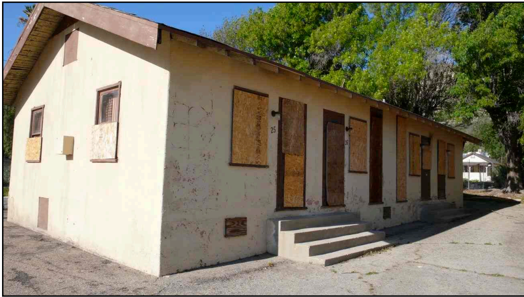
Photo 7. Bunkhouse, southern and eastern elevations [16 February 2008]
