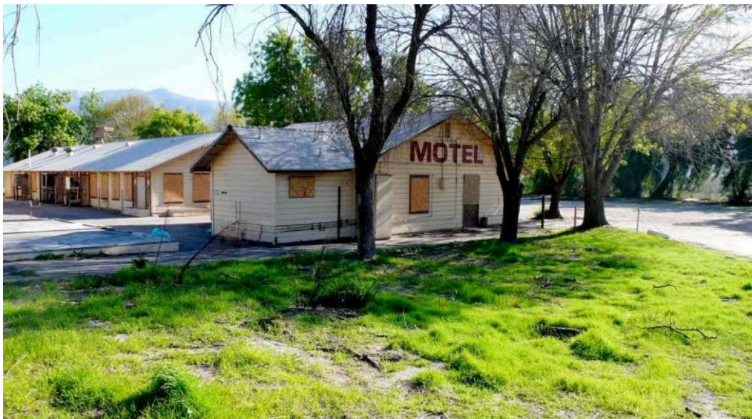
Figure 2 – Office building, northern & western elevations, 2008
