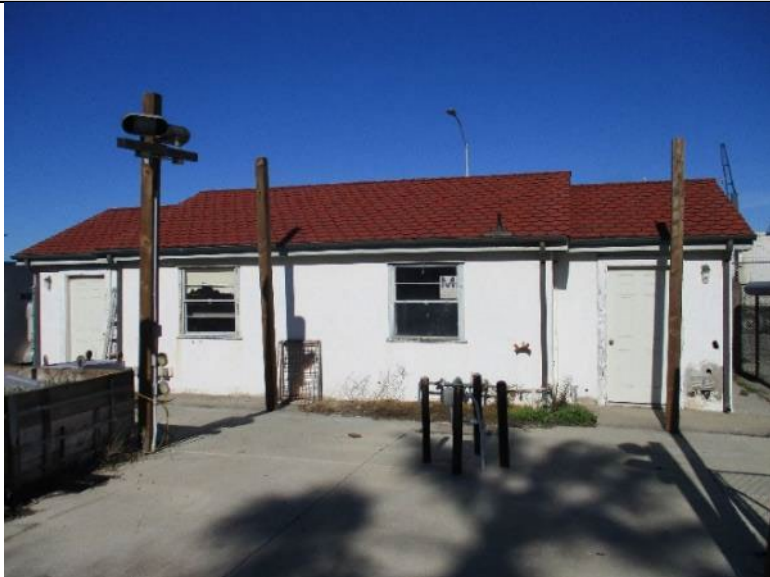
Looking south at the north elevations (IMG_0385)
