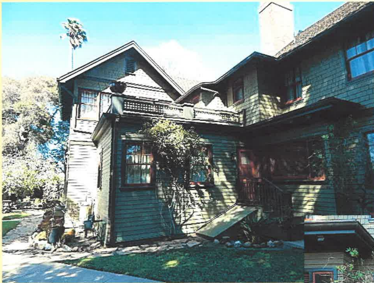
WEST NON-PRIMARY (REAR) ELEVATION SHOWING CELLAR DOOR, SMALL EXIT DOOR, AND MAIN EXIT DOOR TO THE BACK YARD AREA
