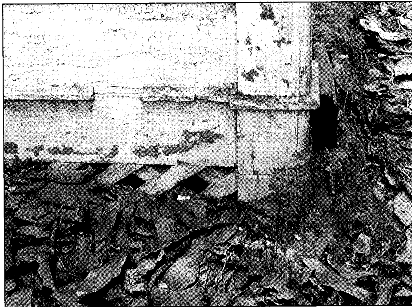
Figure 24. Latticework skirting around the base of the house.
