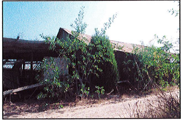
Figure C.14. Ancillary wood barn, ca. 1915, located to the south of the storage area in the Ancillary Barns/Storage Building Group. This view is facing southeast, toward the north and west (primary) elevations. Photograph date, November 5, 2002.
