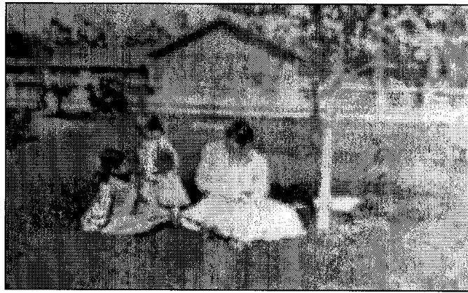
Figure 32. Historical view of barn/garage. (Courtesy of Susan Brown.)
