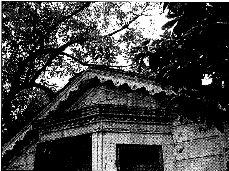
Figure 23. Detail of decorative bargeboard and windows.
