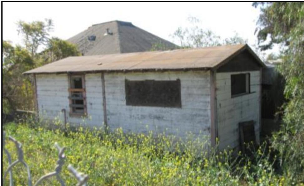
Guest house/bunkhouse situated to the immediate northeast of the main house. View looking southeast. One of the original Victorian-era windows is on the left hand side of the north elevation, while one of the new, unfinished openings is visible in the upper façade of the west elevation.
