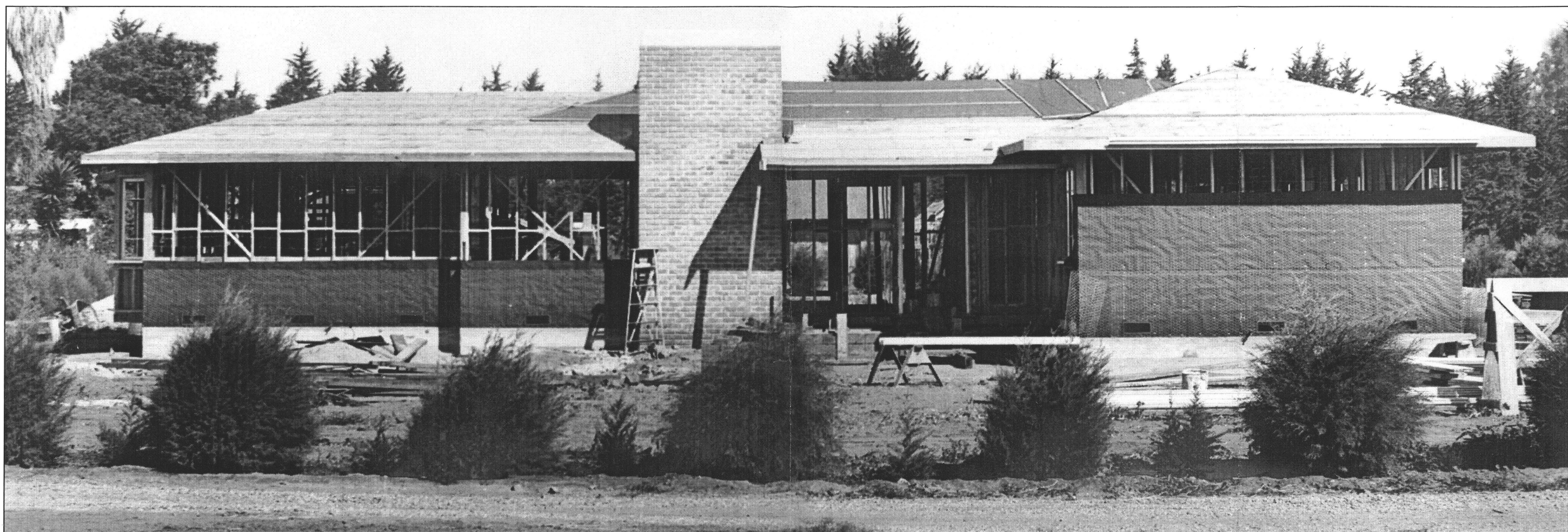
Figure H6. South elevation, ca. October 1948, looking north. The chimney has been completed, and installation of roofing and insulation are underway.
