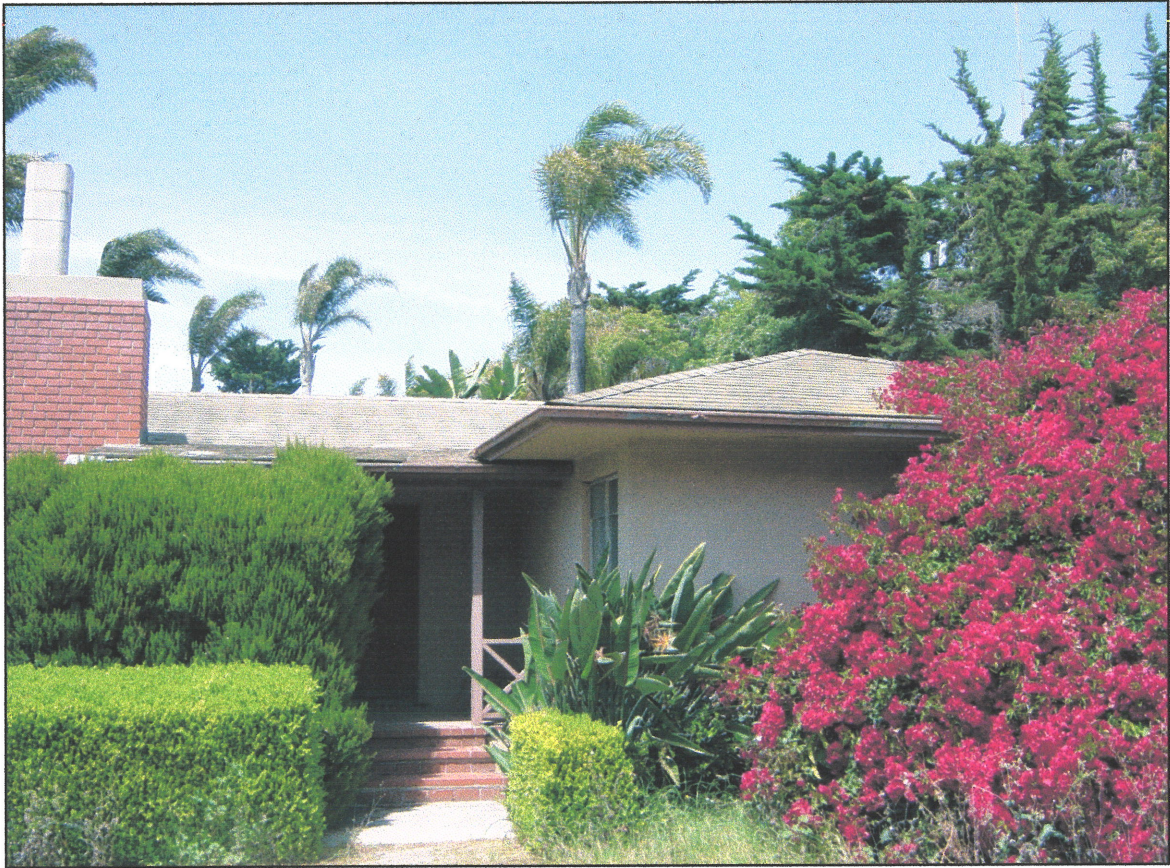
Figure 49. Front entrance on the south elevation of the house. Note the 4-by-4-inch column with an "X" pattern in the railing. The entry has three brick riser stairs. The underhang of the eaves is stuccoed.
