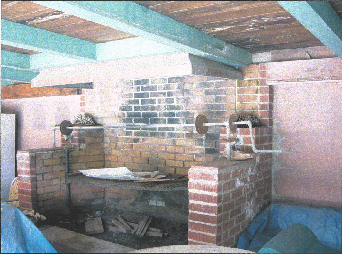
Figure 54. Interior of the BBQ house looking northeast. The brick barbeque is about 6 feet wide with a metal hood. The beams are painted, and the decking is sealed with a natural stain. Infill is 8-by-8-by-16-inch Cement Masonry Units.
