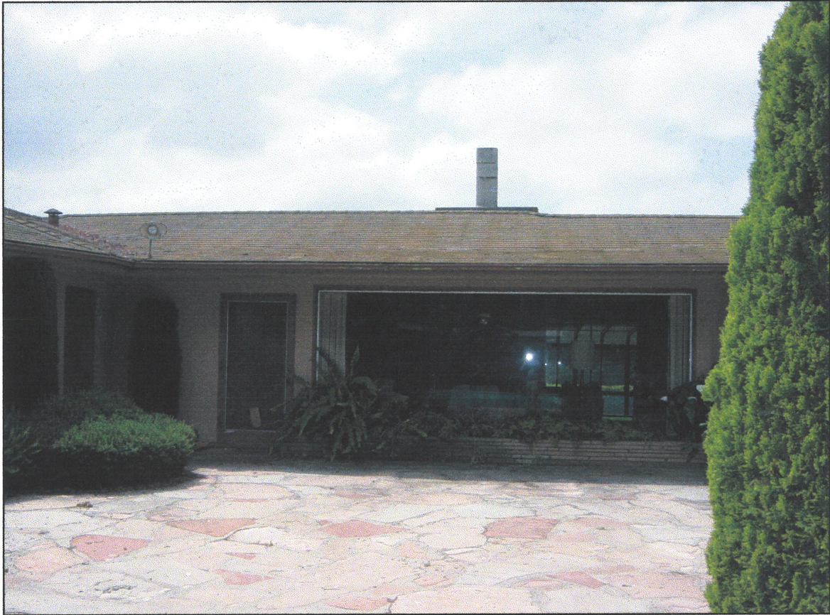
Figure 43. Standing on the patio looking toward the north elevation of the central portion of the house. Note flagstone planter in front of living room window. Door on left opens to entry hall (see Figure 29). The patio is made from multicolored flagstone set in cement mortar, with ~2-foot-wide joints. The chimney extension is visible on the roof to the right of center.
