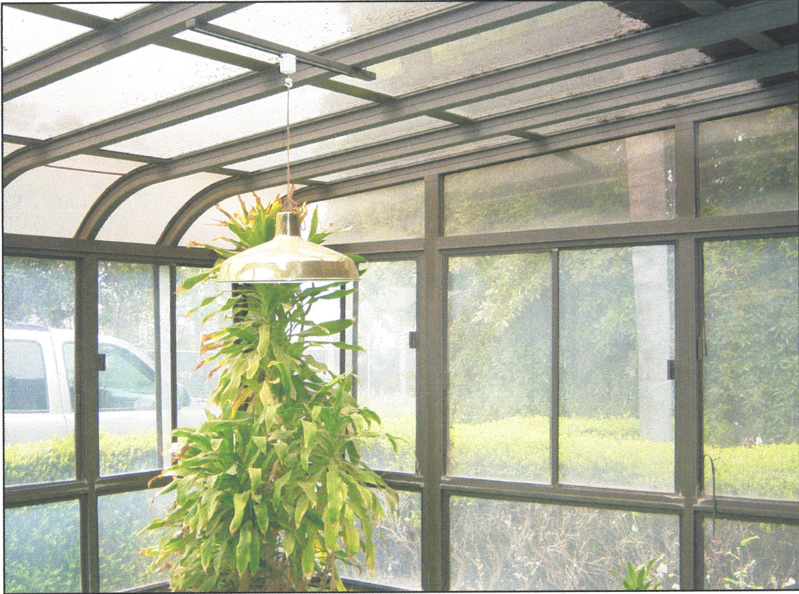
Figure 31. Sunroom with anodized aluminum framing, looking southwest. The sunroom was added on to the southern part of the house in the late 1980s.
