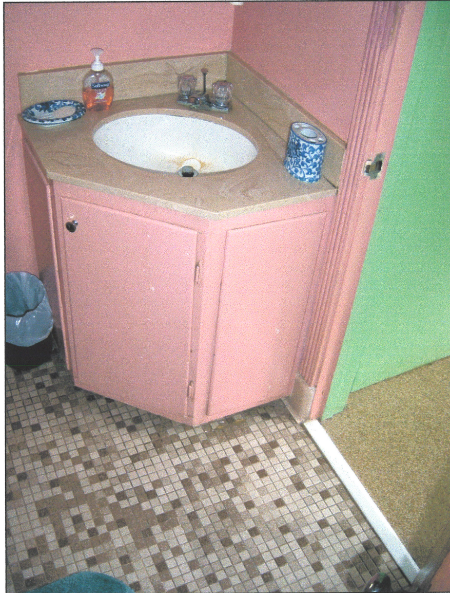
Figure 16. Boys' bathroom looking northeast. The painted cabinet has a recent counter top, sink, and faucet. The floor base is 4-inch nominal with bull-nosed top and cove as well as integral corner-wrapping door frame.
