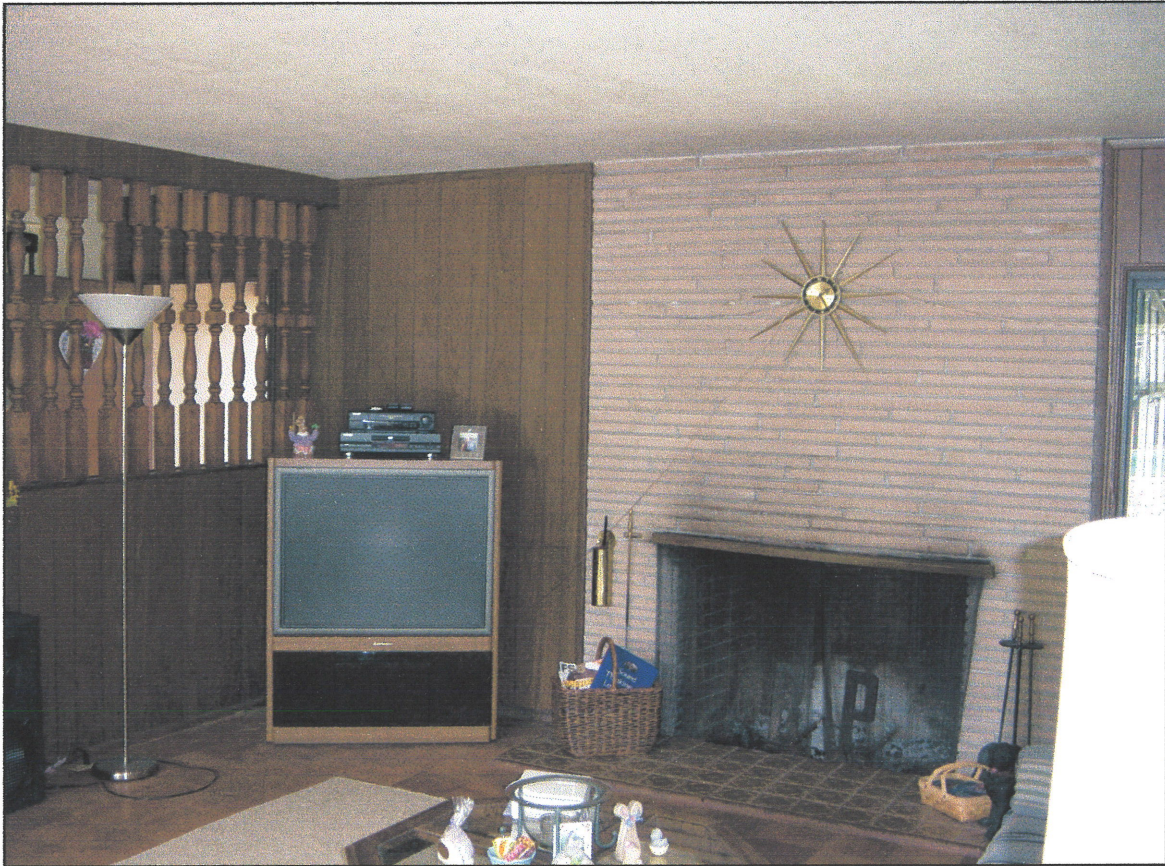
Figure 6. Living room looking south. Flagstone fireplace laid with 1-inch-thick edge exposed. Firebox is fire brick on running bond with a ceramic tile hearth. A wood-paneled half wall with spindles on top to the ceiling separates the entry to the east from the living room. Note original 1950s-style clock.
