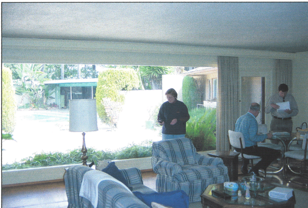
Figure 2. Living room window looking north. This is an exceptionally large sheet of glass, rare by modern standards. Modern code requires tempered glass to be used this close to the ground. The glass is installed in an aluminum frame with screwed-in aluminum stops. The surround and the sill have fluted trim. The existing oak base and oak parquet floor tile are visible. The line of a previous taller base board is visible parallel to the top of the base. Blue paint is visible beneath the yellow paint. Plaster on the walls of the room is smooth with some wicked moisture that caused salt damage at the base of the wall.
