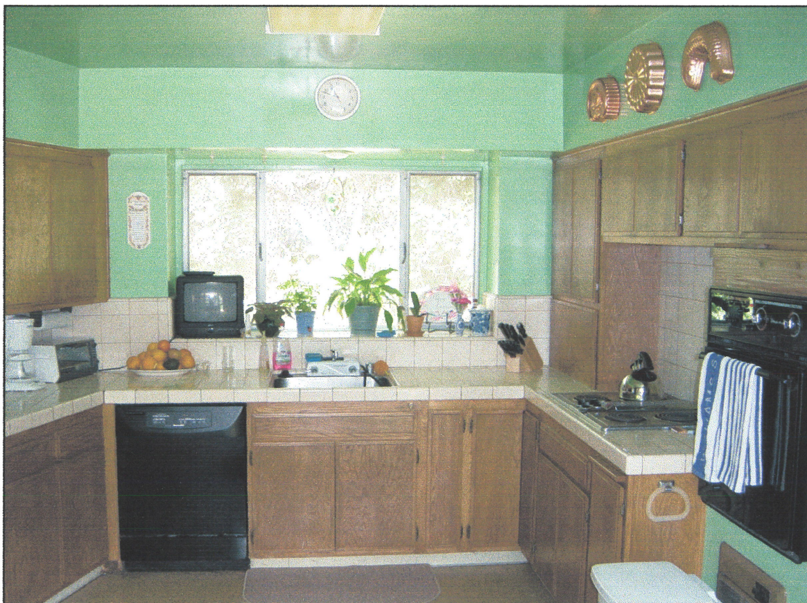
Figure 8. Kitchen looking west. The walls have a smooth plaster finish with semigloss paint. Windows are aluminum, and the counters are made from 6-by-6-inch tiles.
