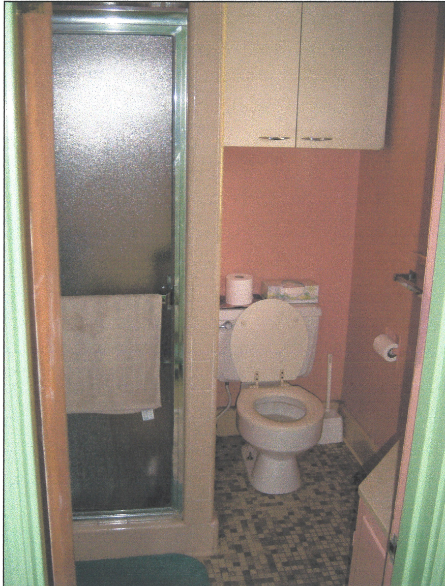
Figure 15. Boys' bathroom looking west. Cabinets are painted wood, and the floor is covered with 1-by-1-inch ceramic tiles. The plaster-and-frame shower enclosure has 4-by-4-inch nominal ceramic tile.
