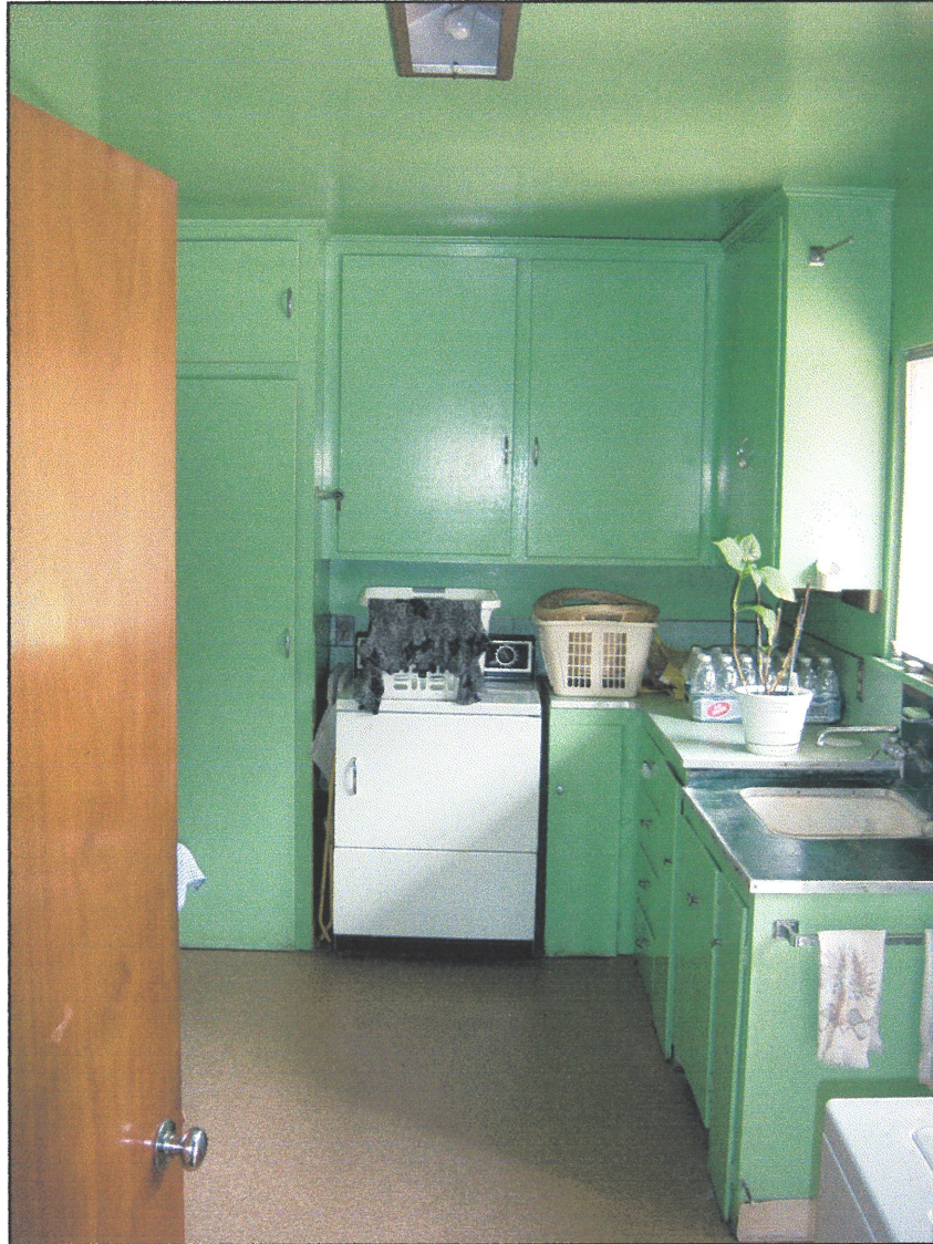
Figure 14. Service porch looking north. Cabinets are painted hardwood cabinets, and there are a birch door and window to the east. Counters are covered with a sheet material held in place with metal trim. The ceiling fixture is recessed.
