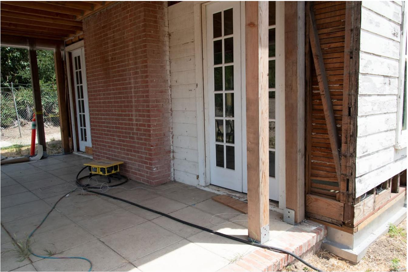
**Figure 20, West Elevation, detail of veranda , existing conditions**
