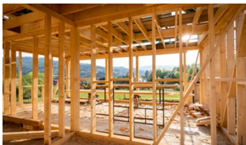
Example of wood framed construction
