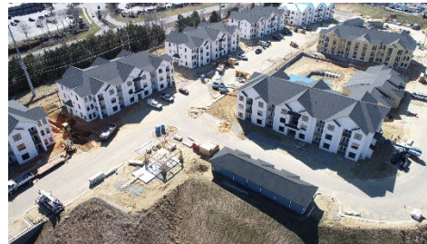
Figure 36. Bulk housing development in North Carolina
