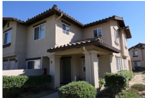
Figure 43. River View townhomes is an 80-unit permanently affordable rental housing provided by People's Self-Help Housing 60
