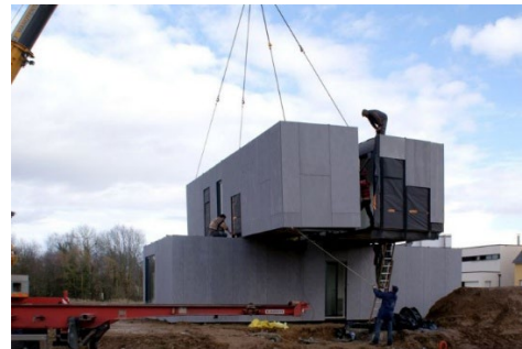
Figure 35. CG Architectes, Crossbox, Modular Housing, construction in progress
