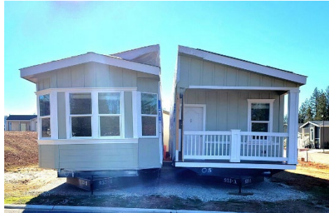
Figure 52. A manufactured home being assembled in Grass Valley, CA.
