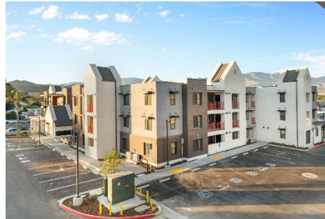
Figure 44. People's Place Apartments in Santa Paula, CA 61
