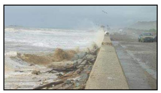
Photo 2-5. This seawall is a form of coastal armoring that is located along the Rincon Parkway. Photo taken during a large wave event (source: D. Revell).
