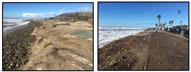
Photo 2-11. The Surfers Point Managed Retreat project (left) after a major winter storm. Downcoast of the managed retreat project (right) storms continue to flood and erode the bike path and parking lot (source: Paul Jenkins).
