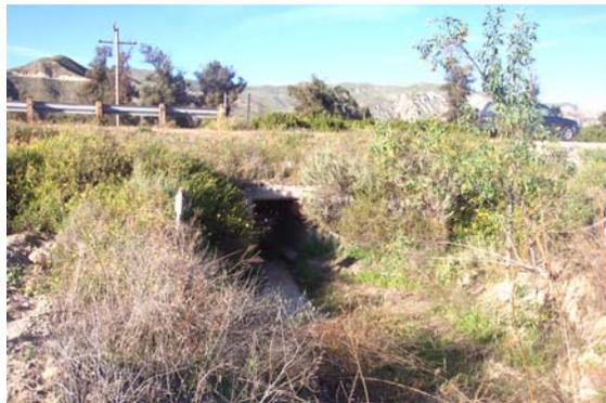
Figure 82. Typical example of concrete drainage culverts.
