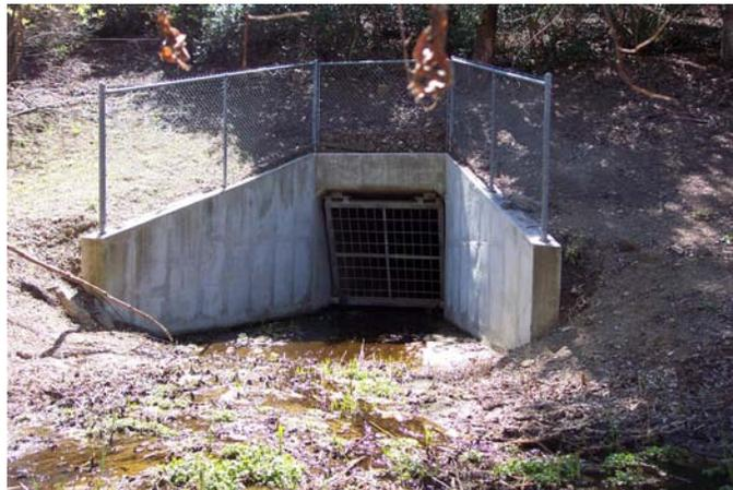
Figure 65. Concrete culvert with trash guard draining Crummer Canyon.
