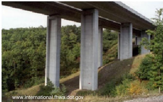
Figure 57. A viaduct in Slovenia built to accommodate wildlife, hydrology, and human connectivity.
