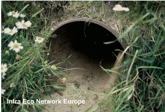
Figure 59. Pipe culvert designed to accommodate small mammals.
