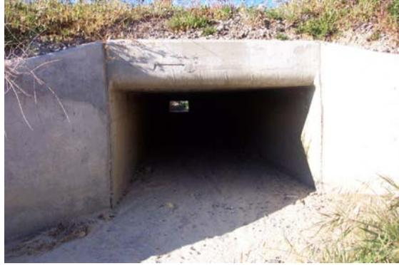
Figure 80. Example of concrete drainage culverts.
