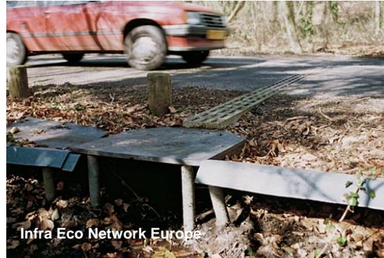
Figure 60. Amphibian tunnels allow light and moisture into the structure.
