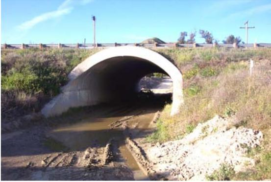
Figure 79. 2-lane arched culvert at Camulos Ranch.
